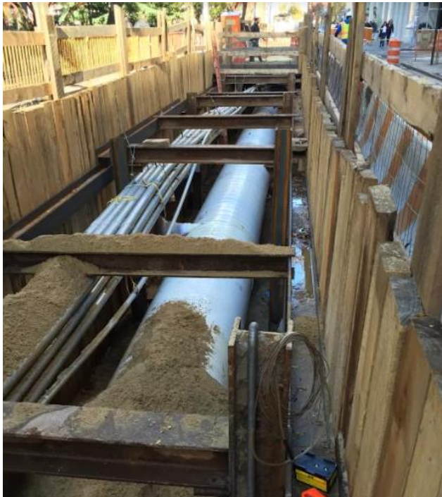
Installation of 48" Trunk Water Main on Washington Sq. East
