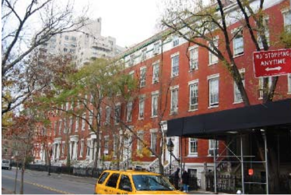
Washington Square North facade
