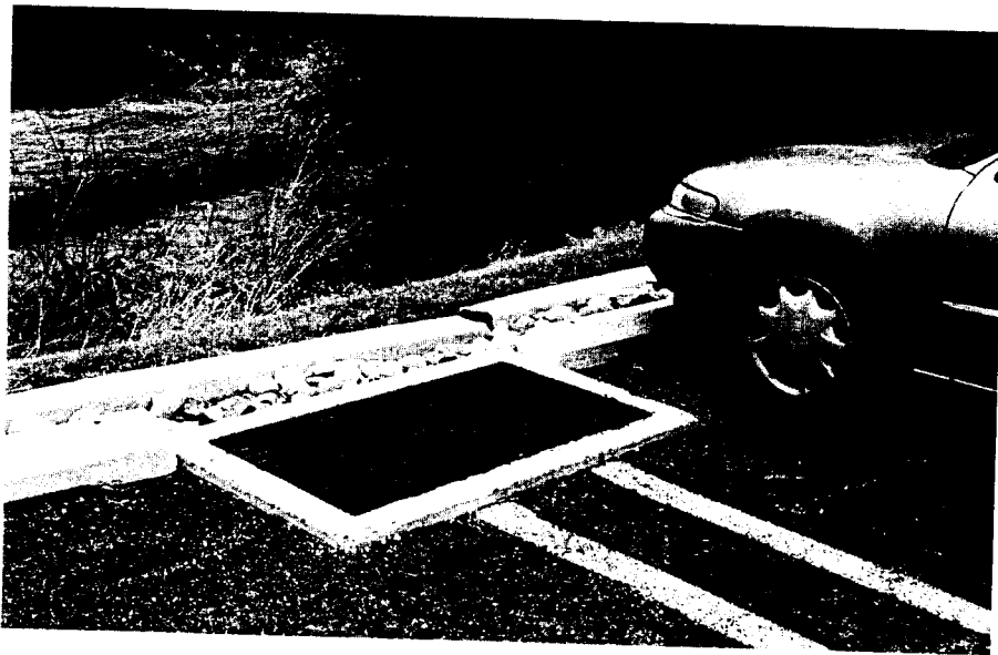
FIGURE 1.17 Porous asphalt parking lot protecting stream water quality at Exton Square Mall in Exton, Pennsylvania.
