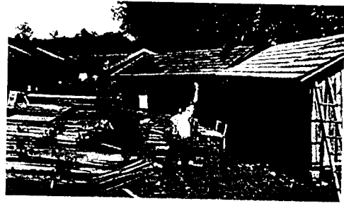
1917 Demountable Wooden House France (various locations) American Friends Service Committee Built by volunteers to house World War I refugees, each "demountable" wooden house consisted of two rooms. American Friends Service Committee
